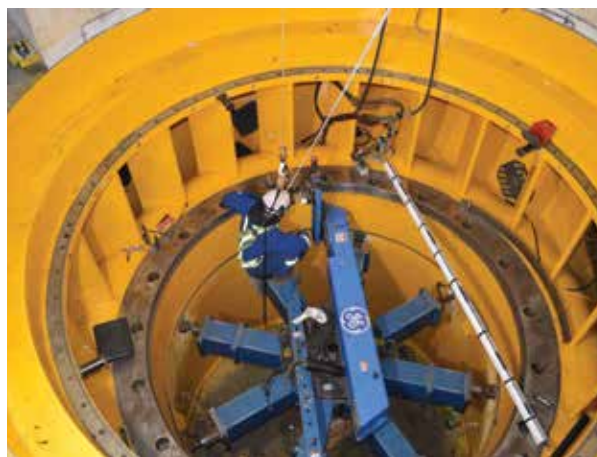
Machining the seal ring on Snare Forks turbine.
