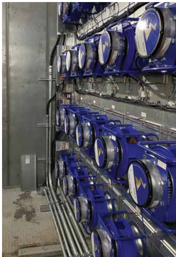
This modular fan wall reduces electricity consumption in Yellowknife's Laing Building.
