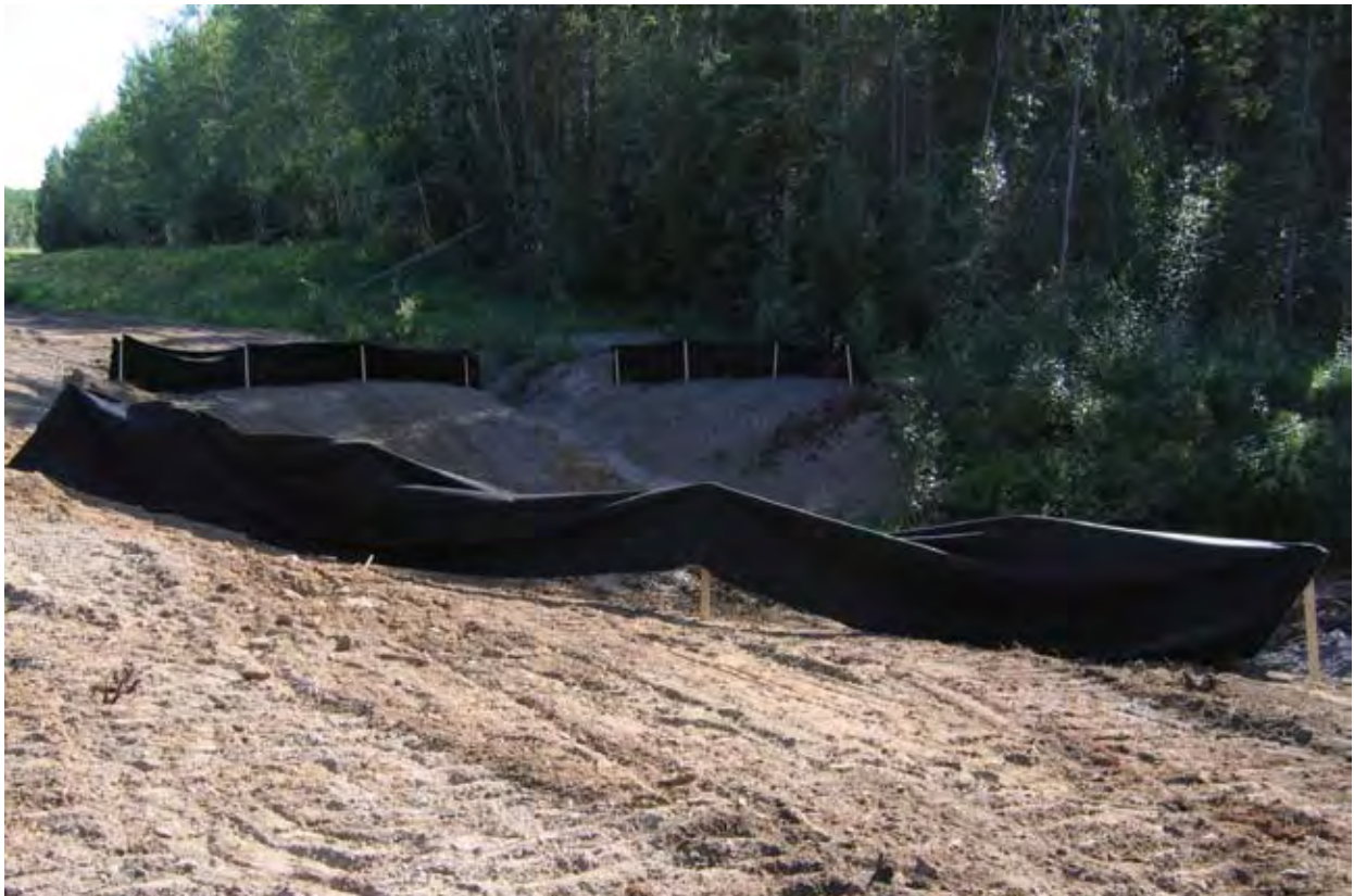
FIGURE 17. Sediment curtains used for drainage control at the edge of a clearing.
