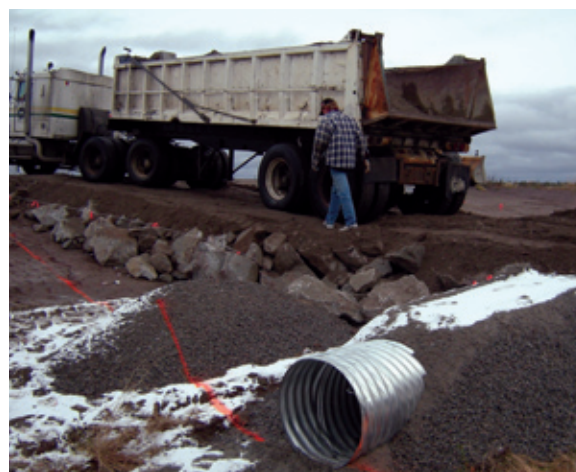
FIGURE 17. This cross drain is covered with coarse-grained granular material for frost protection.
