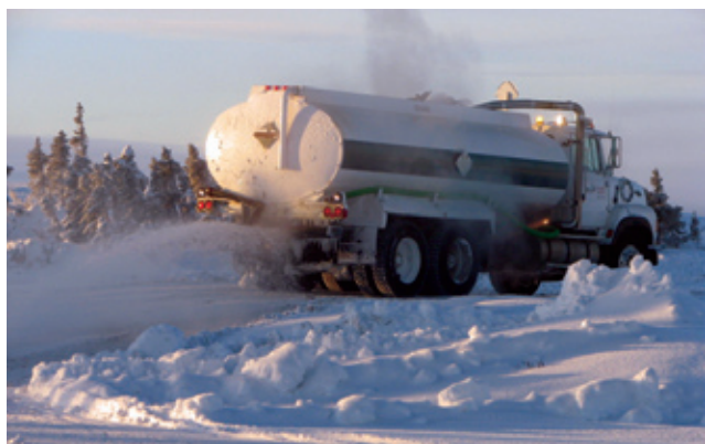
FIGURE 30. The road surface can be built up with ice using a water truck with a sprayer.
