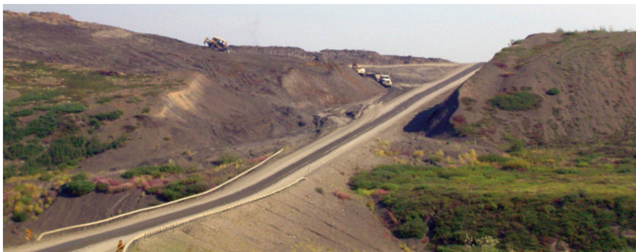
FIGURE 16. The slope of this road has been reduced by fill excavated from the adjacent cut. Drainage and Erosion Controls
