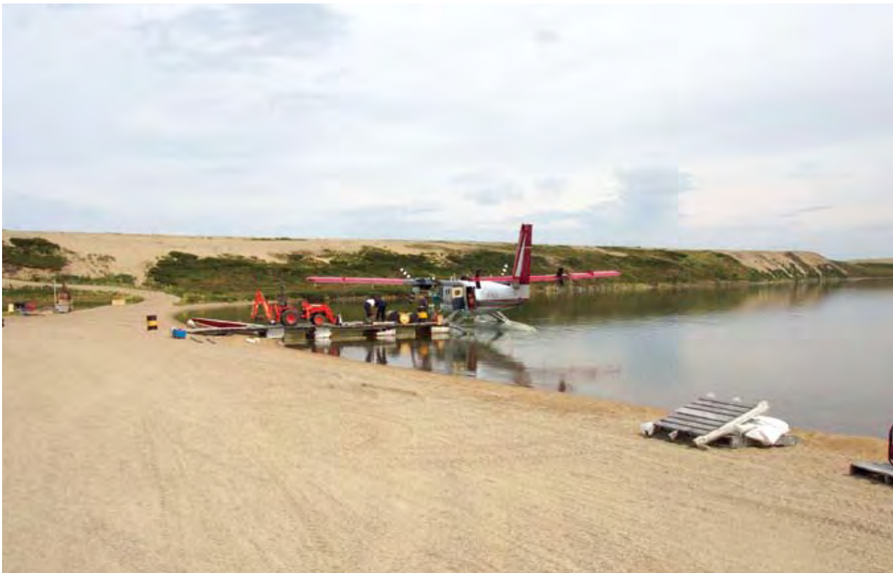
FIGURE 12 (BOTTOM) A dock should be located in a sheltered area with a gentle shore and adequate water depth for float planes and boats.
