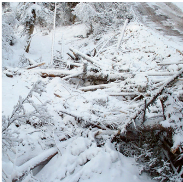
FIGURE 34. A poorly constructed snow fill consisting of mixed brush and snow.
