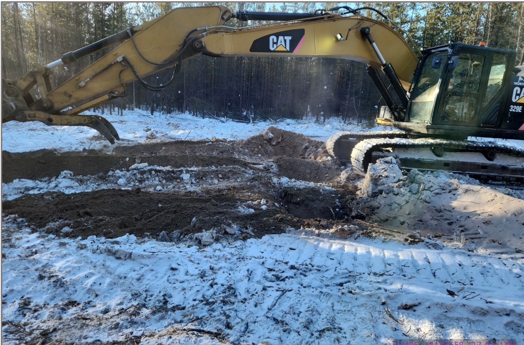
Photo 4: Borrow Source 9.002 (North) Testpitting Backfilling completed for Testpit TP25-9.002-05 (Photo Date: March 26, 2025)
