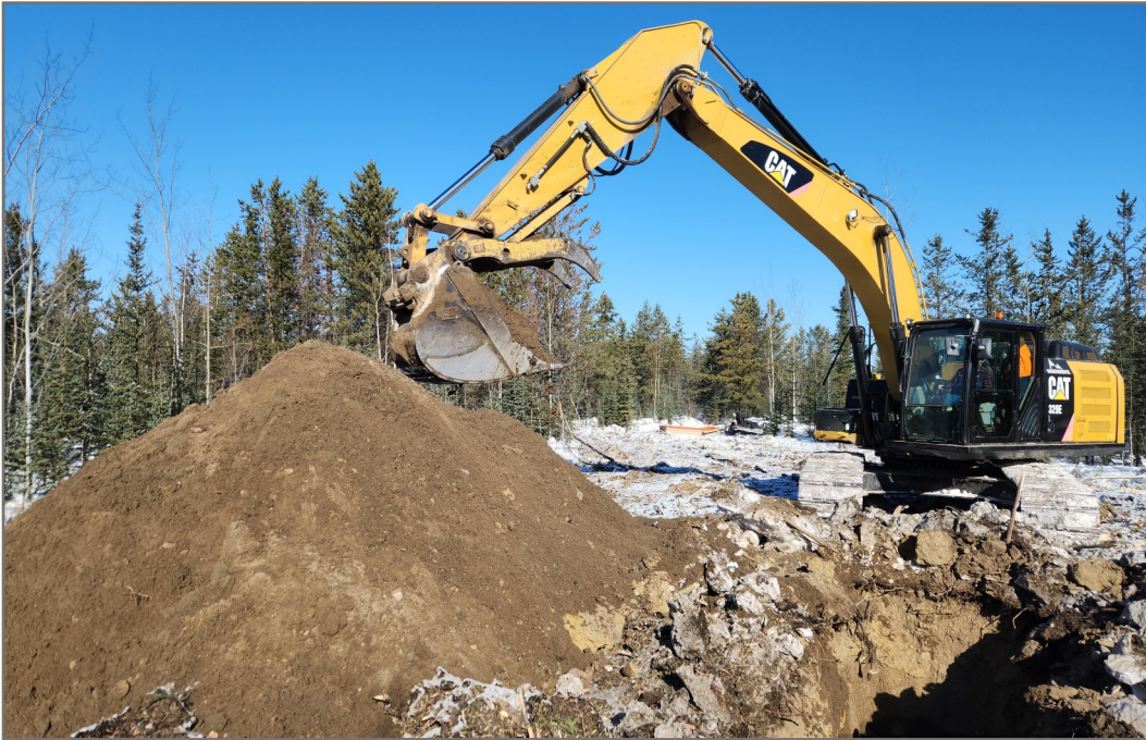
Photo 5: Borrow Source 9.002 (North), Testpit TP25-9.002-01 Sand excavated from Testpit TP25-9.002-01 (Photo Date: March 25, 2025)
