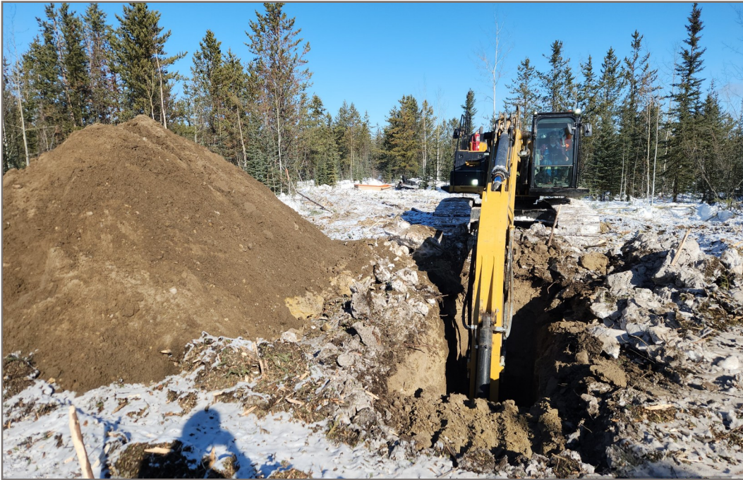
Photo 3: Borrow Source 9.002 (North) Testpitting Excavating for Testpit TP25-9.002-01 (Photo Date: March 25, 2025)
