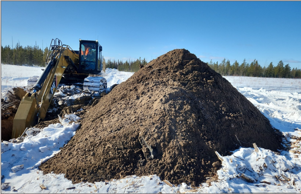
Photo 7: Borrow Source 9.002 (North), Testpit TP25-9.002-02 Gravel and Sand excavated from Testpit TP25-9.002-02 (Photo Date: March 25, 2025)
