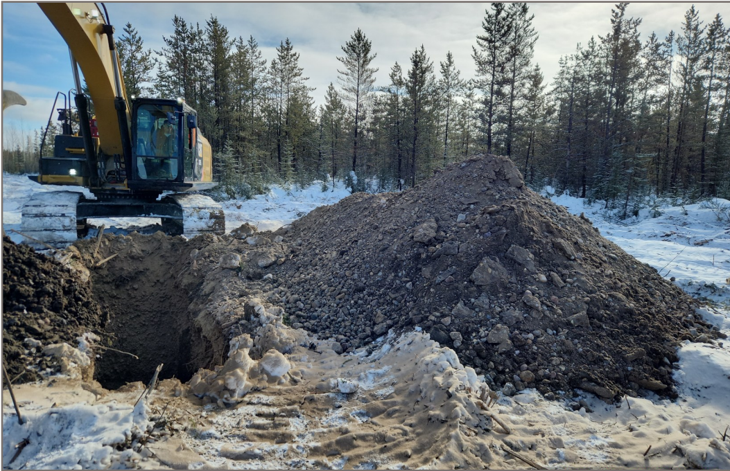
Photo 15: Borrow Source 9.002 (South), Testpit TP25-9.002-06 Gravel and Sand excavated from Testpit TP25-9.002-06 (Photo Date: March 25, 2025)
