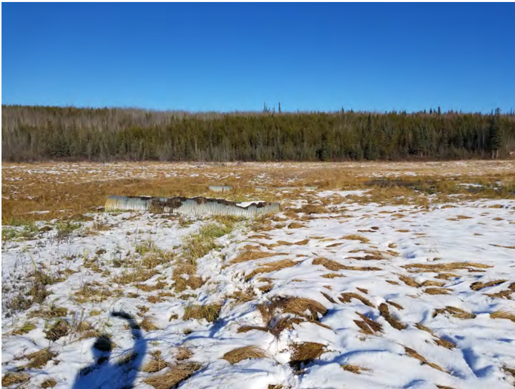
Photo 6: Site 820.7—Damaged culvert at existing centerline.
