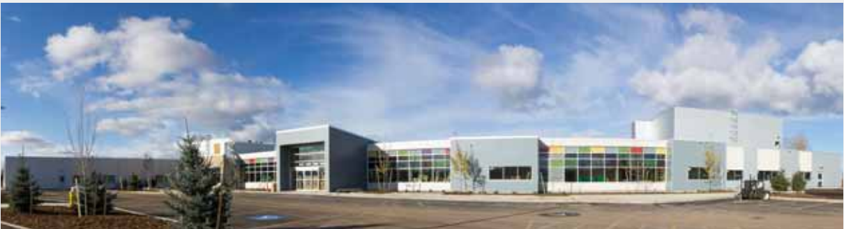
The new Hay River Health Centre
