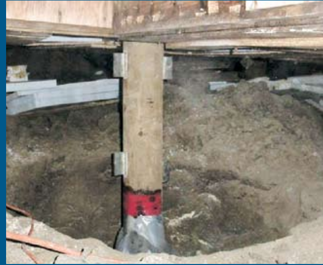
The rotted portion of this pile has been replaced with new material.
