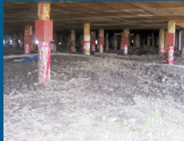
Steel sleeves connect new piles to solid portions of original piles.
