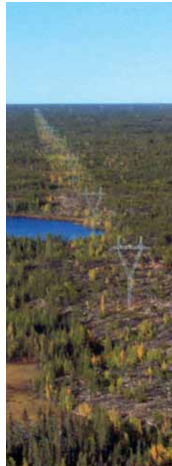
A row of transmission lines.
