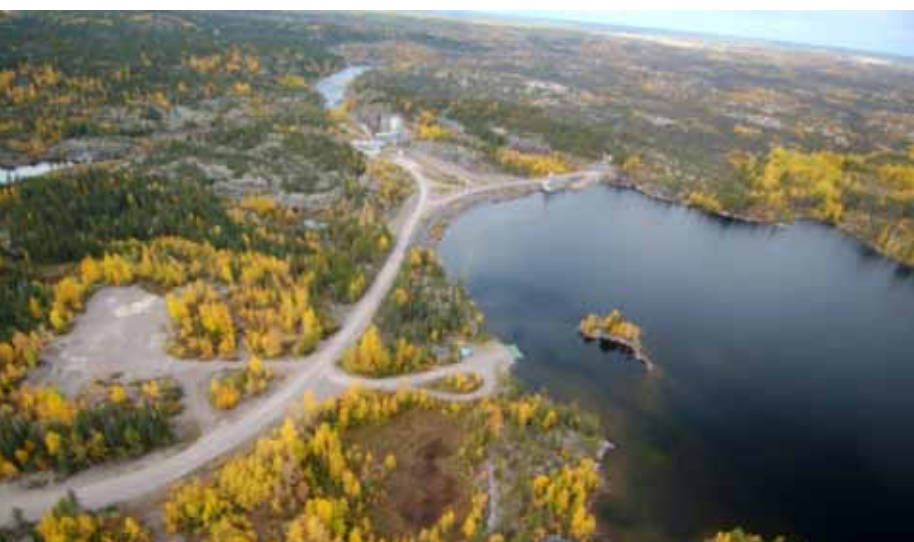
An aerial picture of the Taltson hydro facility.
