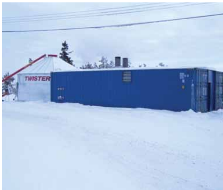
A wood pellet facility in Yellowknife that provides heat to a building as an alternative to diesel fuel.
