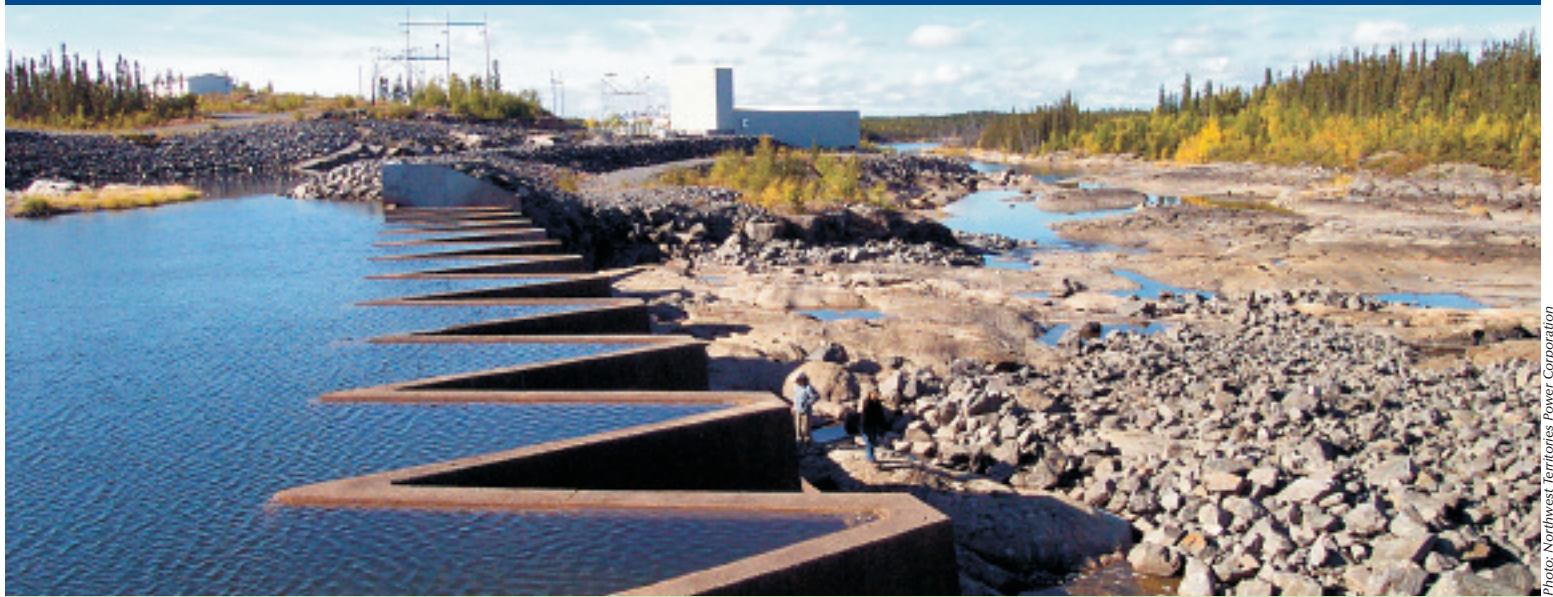
Snare Cascades Spillway
