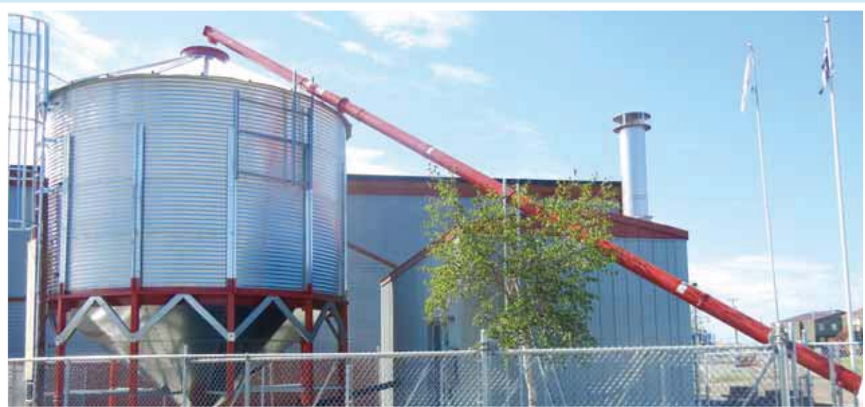
Elizabeth Mackenzie Elementary School – Wood Pellet Boiler installation
