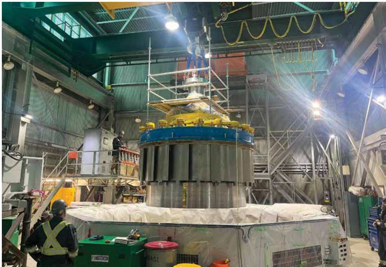
Generator being installed
