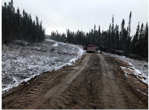
Construction underway on the Austin Lake Access Road in Łutselk'e.
