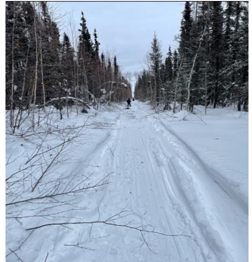
Access trails continuation construction - Nahanni Butte.
