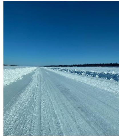
Driving along the 80KM Fort McPherson section of the Peel River Ice Road constructed from Fort McPherson to the Esau Creek midway point.
