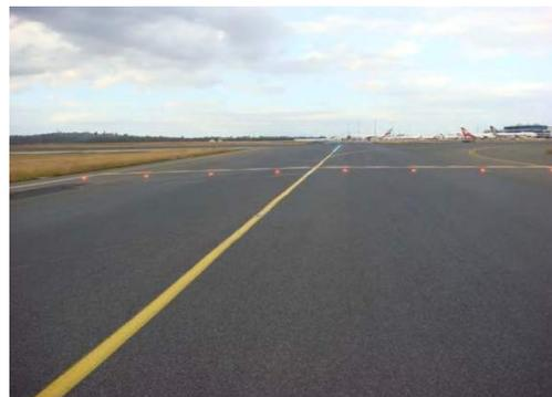
**Taxiway Centre Line Marking** - Some airports will outline the yellow lines with black lines in order to increase the contrast between faded pavement and the yellow lines. When the pilot centers the aircraft nose wheel on the line, it helps to ensure the aircraft wheels will remain on the paved surface and the aircraft wing tips will not come in contact with an obstruction.
