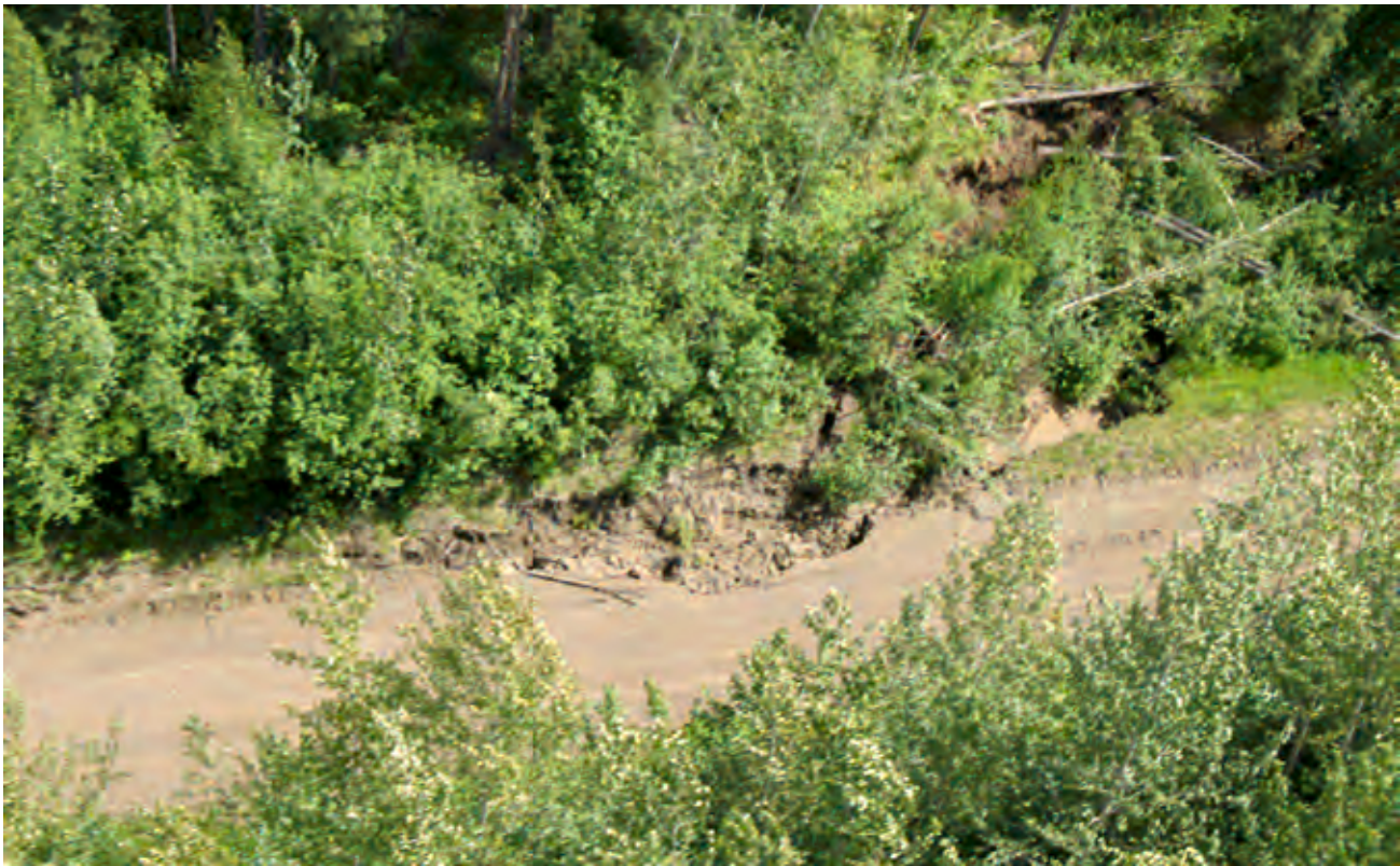
FIGURE 37. Regular monitoring will identify areas prone to erosion that may need to be redesigned.
