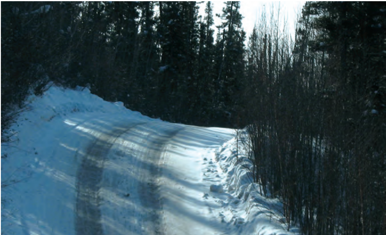
FIGURE 6. Road grades and curves should be designed to be safe and minimize environmental disturbance. In this case, a wider curve and a lower grade would be safer and less prone to erosion.
