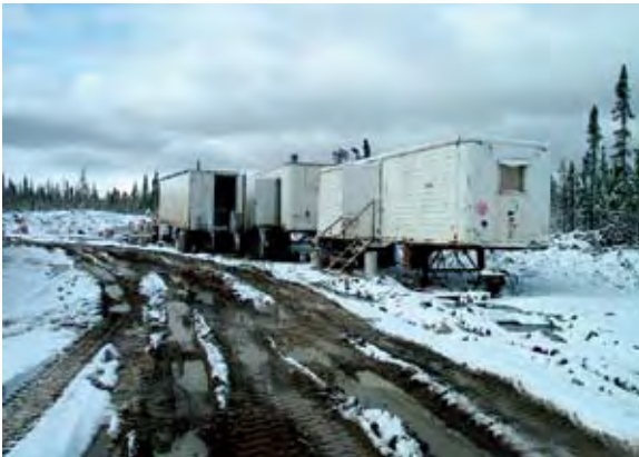
FIGURE 13. Deep rutting and soil erosion can occur if operations continue too late in the spring.
