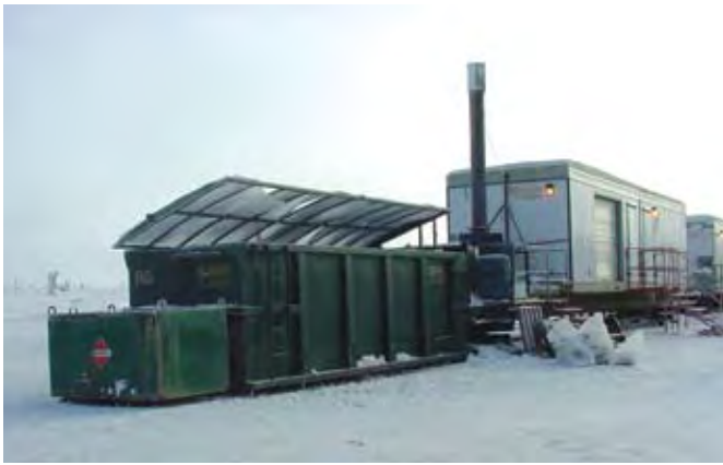
FIGURE 20. A fuel-fired incinerator with a bin nearby to store non-combustible wastes.
