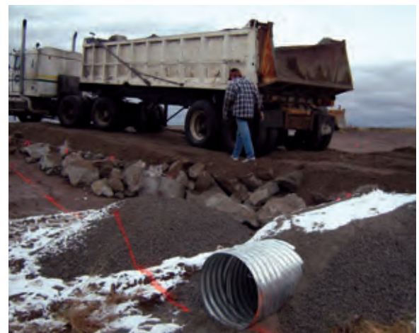
FIGURE 17. This cross drain is covered with coarse-grained granular material for frost protection.
