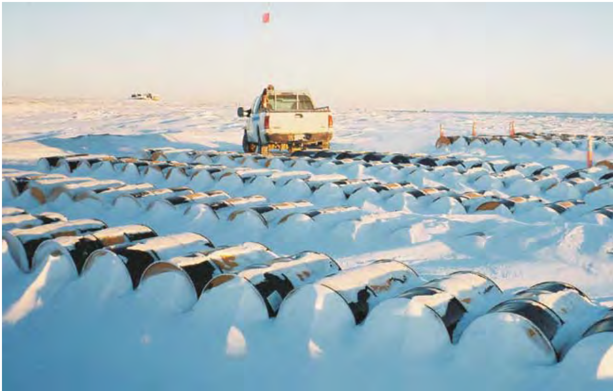
FIGURE 19. This fuel storage area is well marked with pylons, and drums are stored on their side and well spaced to allow for leak inspection, but snow should be cleared to facilitate leak inspection.
