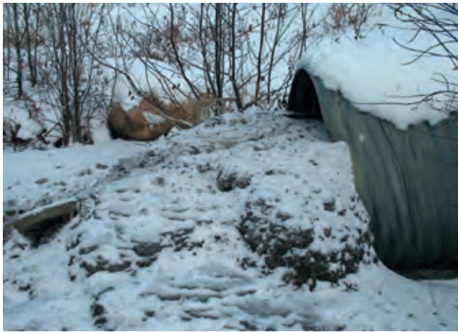
FIGURE 38. Culverts should be monitored and cleaned regularly to ensure that they continue to function properly.
