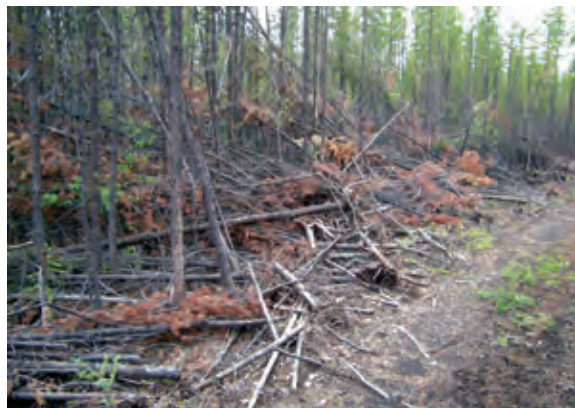
FIGURE 15. Improper disposal of brush in forest vegetation. Leaners should be cut down and brush windrowed.
