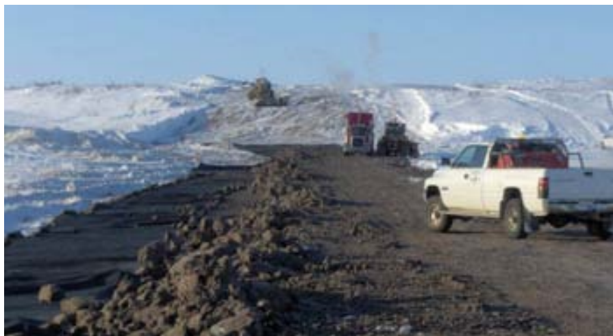
Photo 2.6.3-2 The winter construction approach; note the grader in the distance clearing snow from the embankment footprint. (Tuktoyaktuk to Source 177 Access Road, 2009)
