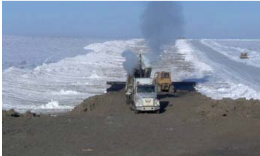
Photo 2.6.3-1 An example of winter road access constructed parallel to the road (Tuktoyaktuk to Source 177 Access Road, 2009)
