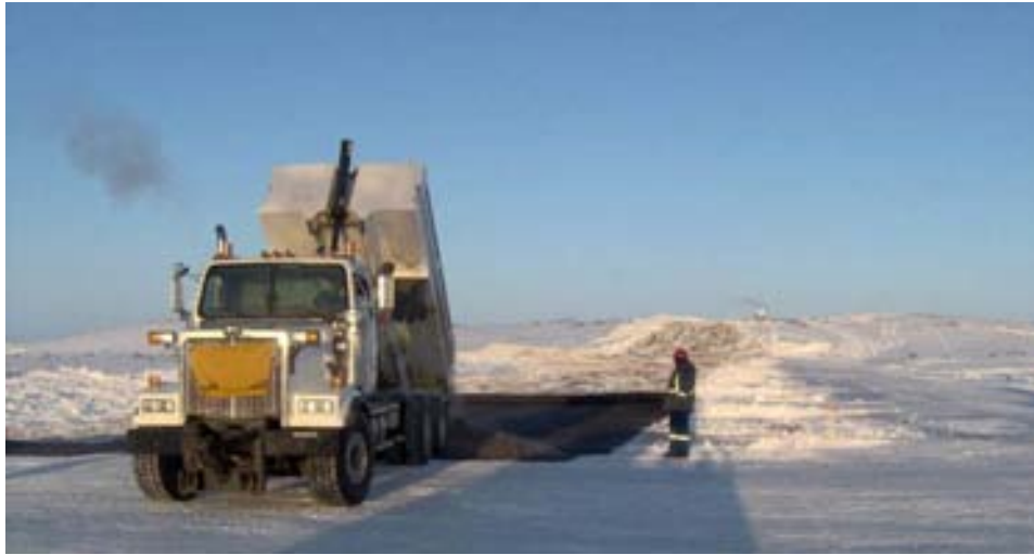
Photo 2.6.3-3 An example of geotextile placement and the proposed end-dumping method of construction. (Tuktoyaktuk to Source 177 Access Road, 2009)
