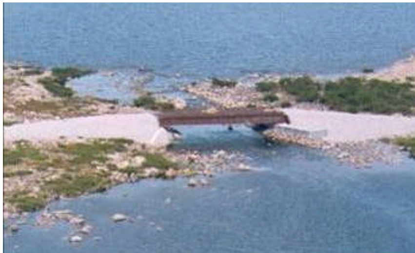
Photo 2.6.6-1 Single span, prefabricated bridge on gravel filled binwall abutments
