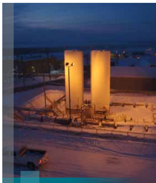
LNG Storage Facilities in Inuvik (Source: GNWT)
